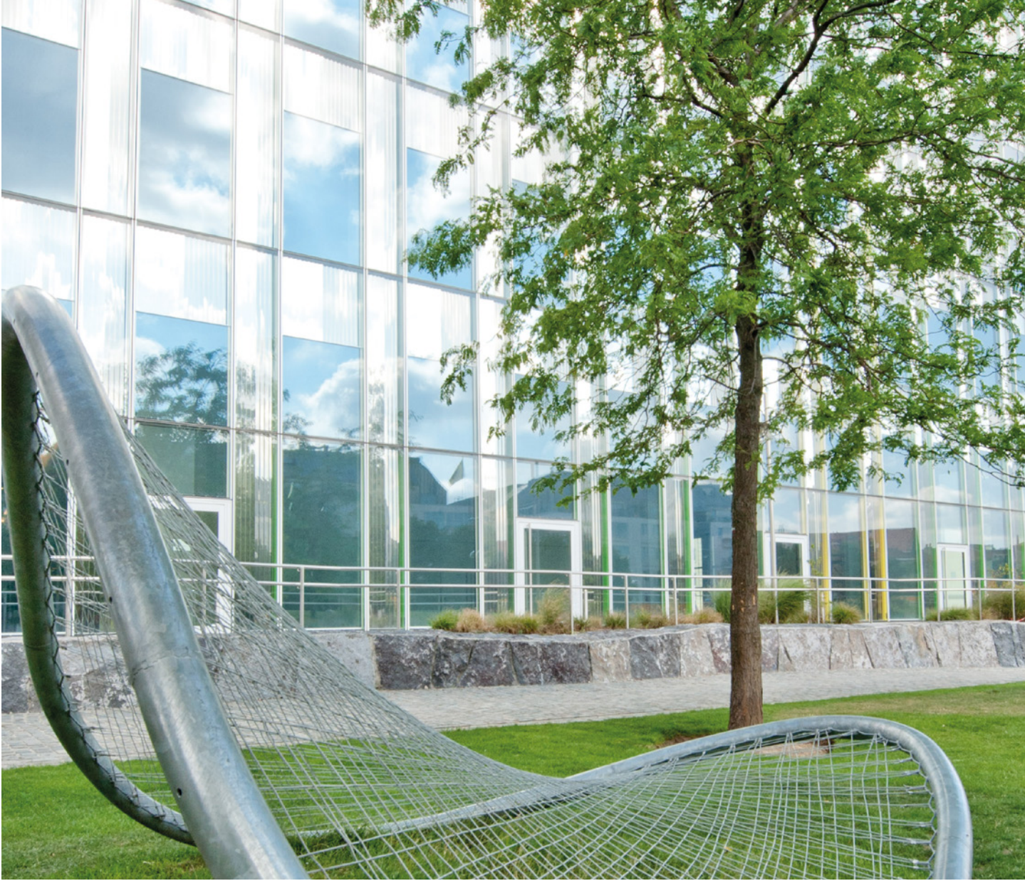
Zenith Building, Brüssel
